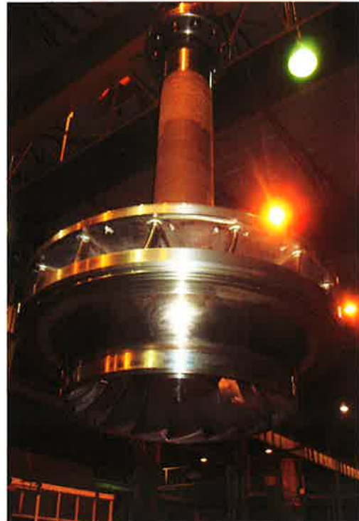
Figure 2 – Guthega Stator Lift
