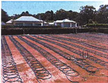
Figure 6: Large horizontal "slinky" ground loop installation before backfilling
