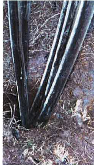
Figure 3: Double ground loops in a borehole with a grout pipe.
